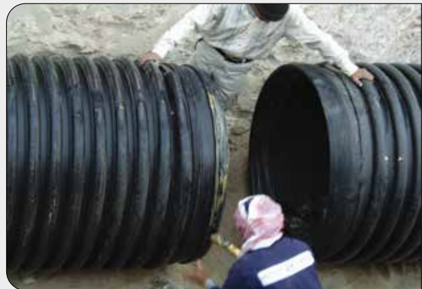
Applying Lubrication to socket and spigot, after cleaning, at Kuwait
