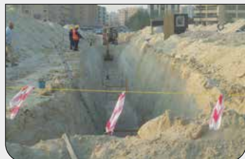
Trenching at Kuwait
