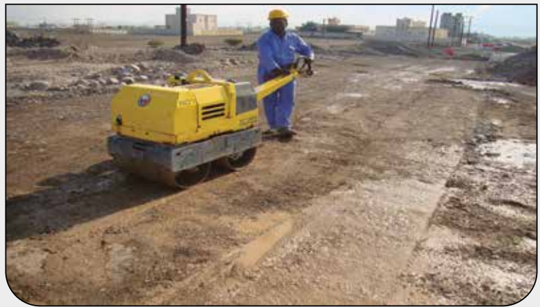
Final Backfill at project in Oman
