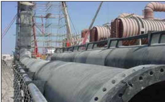
NIC HDPE Corrugated Pipes with flanged connection for sea water intake project in UAE
