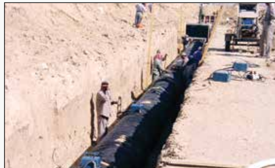
NIC HDPE Corrugated Pipes for Storm Water with electro-fusion connection at project in Kuwait
