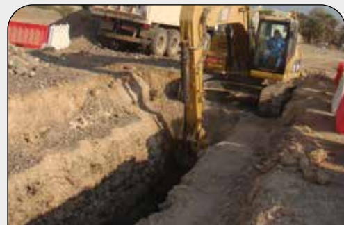
Trenching at Oman
