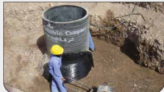
Initial backfill at project in Oman
