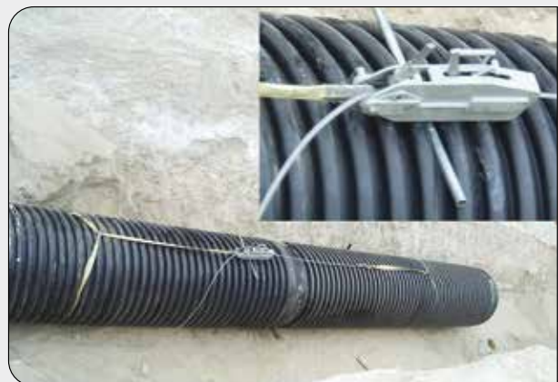
Assembly of pipes at project in Kuwait
